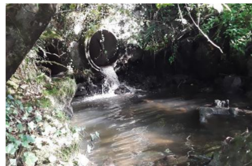
Obstacle infranchissable (buse)
